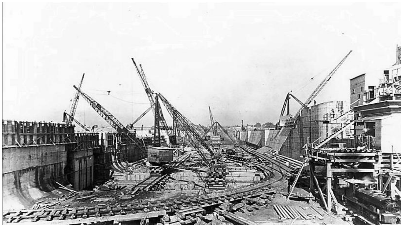
Above: The new graving dock under construction – note railway tracks and locomotive
